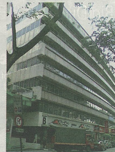
Will Pusat Bandar Damansara see major refurbishment works this year?
